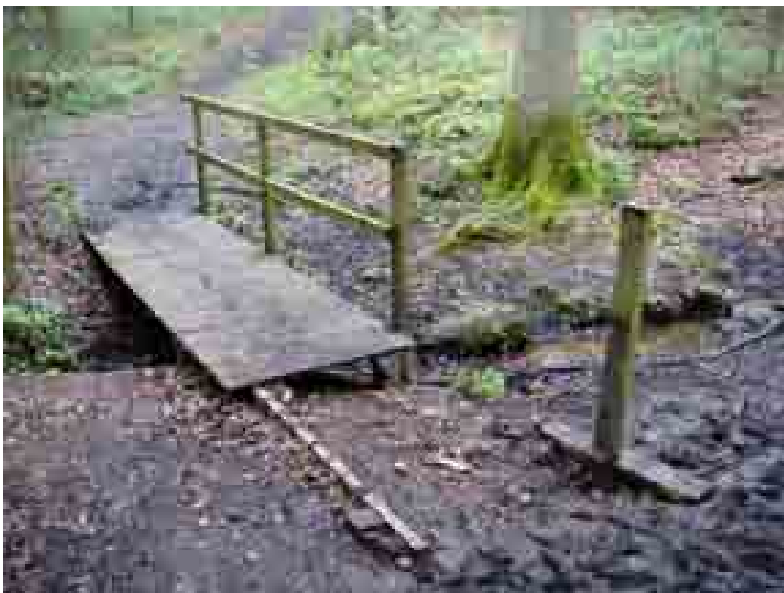
The footbridge as left
